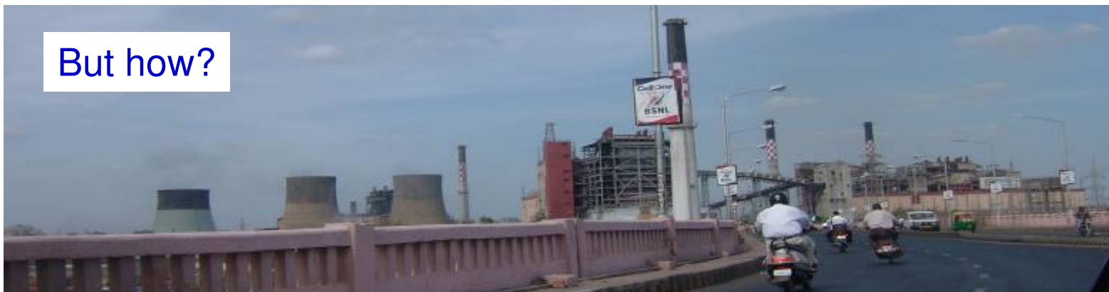
Ahmedabad power station, June 2007
